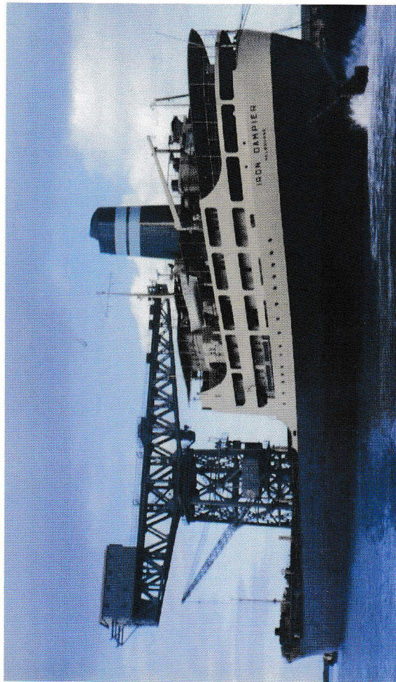
Iron Dampier fitting out at Whyalla in 1960
